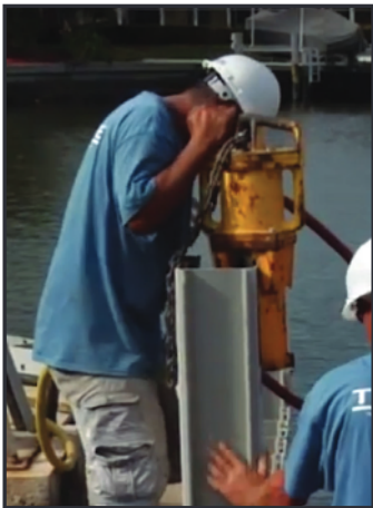
Slotted Master Chuck (P/N 070597) Attached for driving sheet pile.
