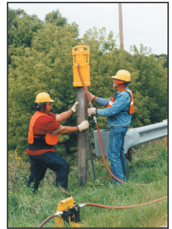
6" x 6" Master Chuck (P/N 070761) Attached for square wood pile.
